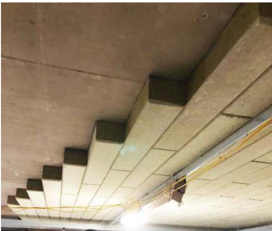
MANCHESTER OFFICE DEVELOPMENT / MINERAL WOOL INSTALLATION
